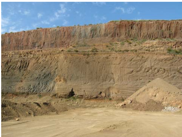
Fig. 2 Sub-vertical cut in a quarry of Pozzolana; from the bottom it is possible to recognise the layers of Pozzolana Nera ( \cong 10 m), Tufo Lionato ( \cong 5 m), and Pozzolanelle ( \cong 8 m)
